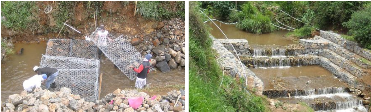
Figure 7. Construction of gully plug by using gabion
