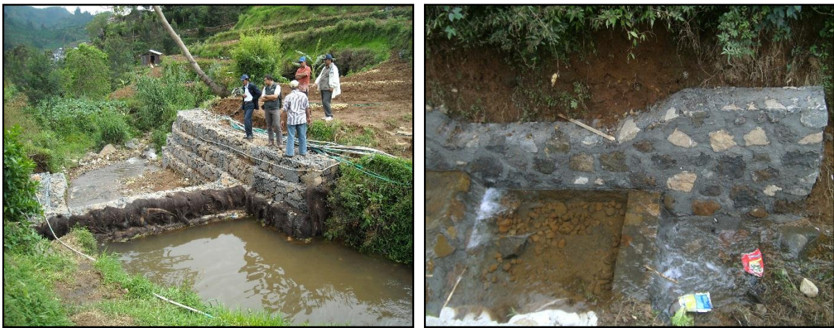
Figure 17. Small dams and gully plug construction
