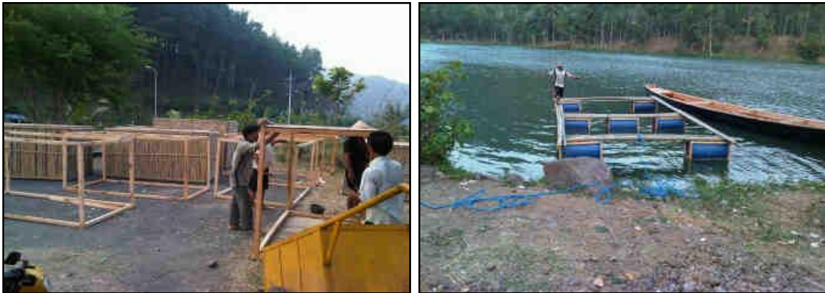
Figure 20. Fish cage construction for Serayu river
