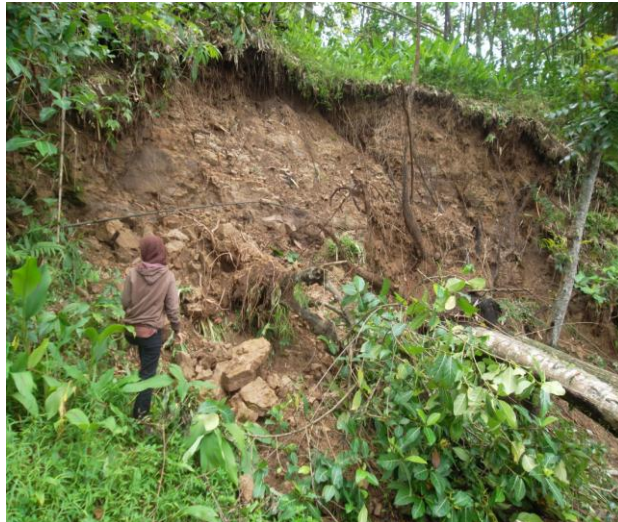
Figure 3 Steep Slope with Lithic Soil
