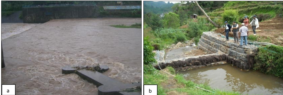
Fig. 5. a). Suspended load on the river, b) ). Sediment control structures
